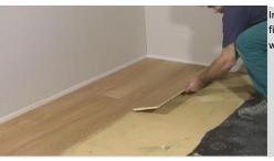
Install the floor finishing (ceramic or wood)
