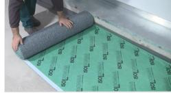
Install the acoustic mat with rubber granules facing down
